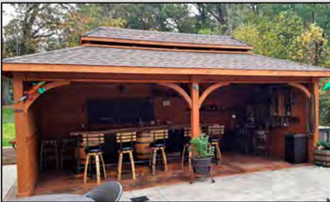
12'x24' · HD braces · custom wall enclosures · extended overhang · dimensional shingles · cedar sealer
